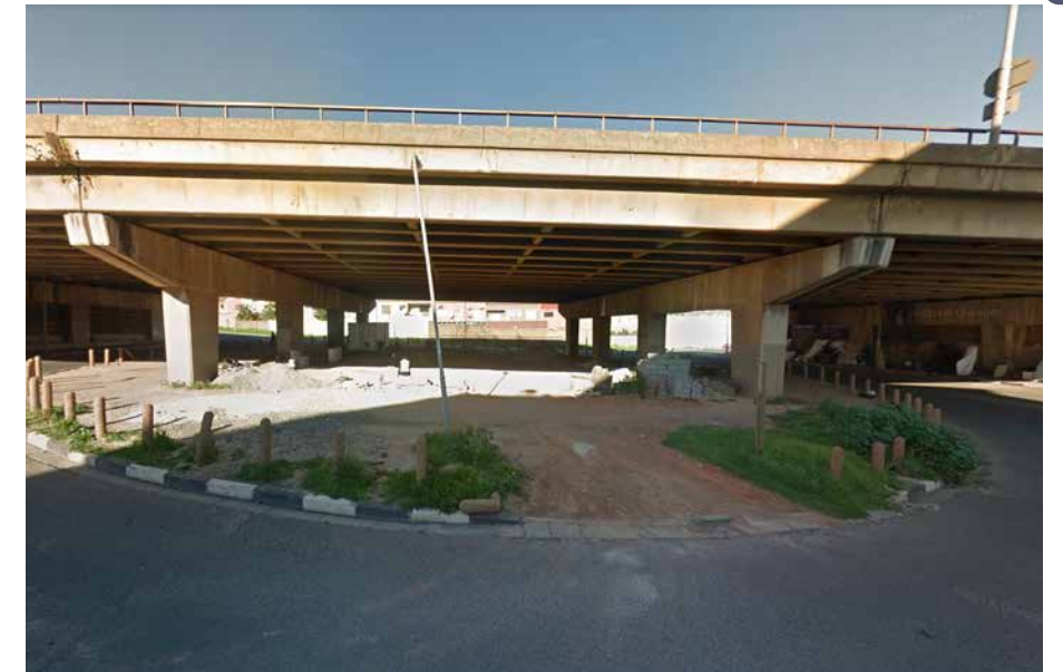
Fig. 5.129. Circle under Highway, Intersection of Chapel Street &amp; Russel Street
